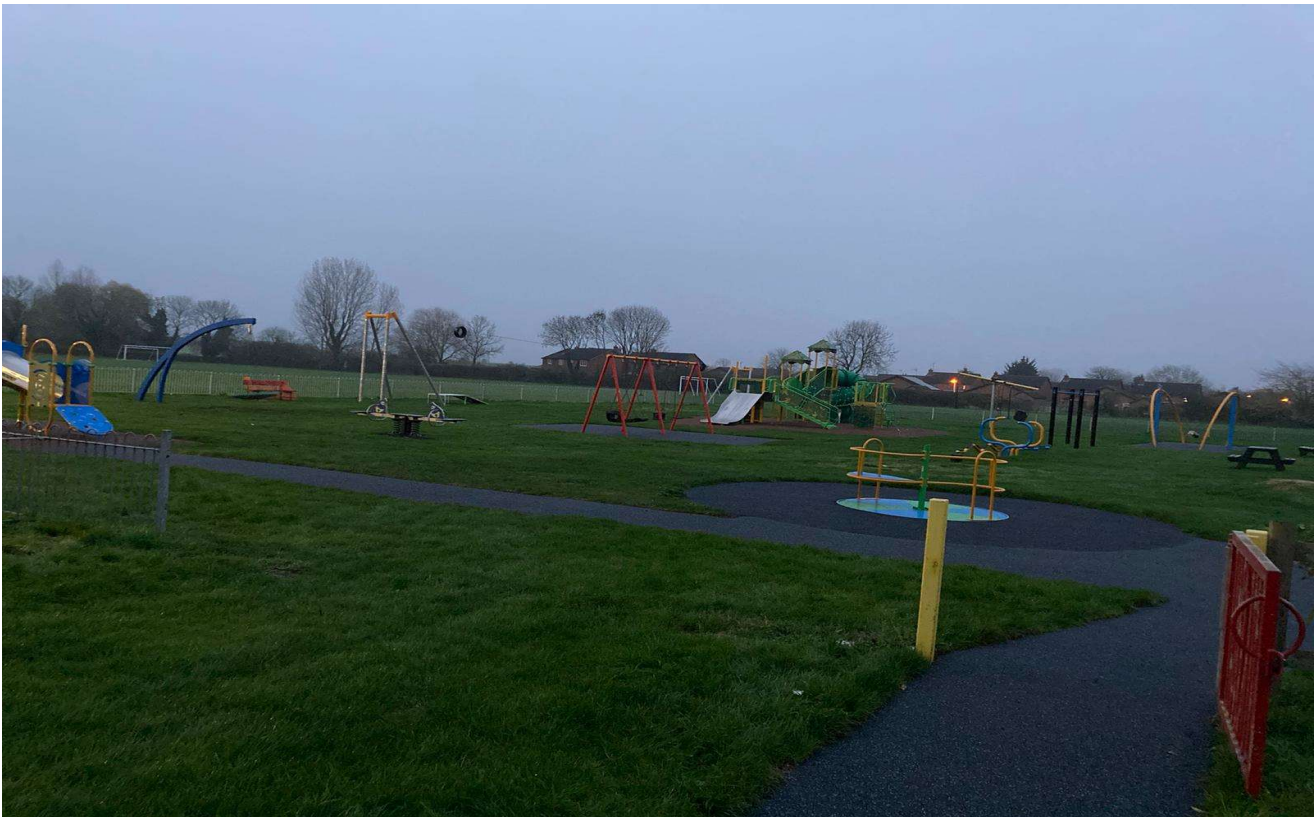
Figure 3 The Completed Play Park Project at Parkfield
